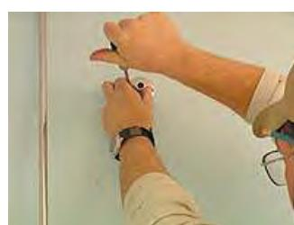
31. Slide the post into the bracket and tighten the set screw.
