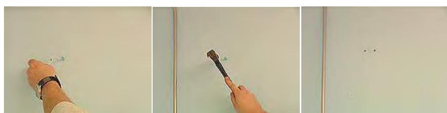
30. Place the screws into the escutcheons and use the screwdriver to screw into the anchors in the wall.
