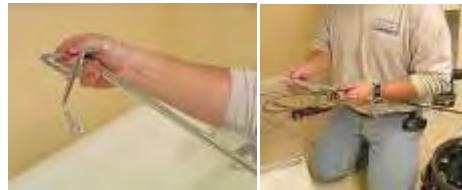
18. Take the locknut from the diverter valve and place it at that bottom of the riser pipe. Slide the friction ring and washer onto the bottom of the riser pipe.
