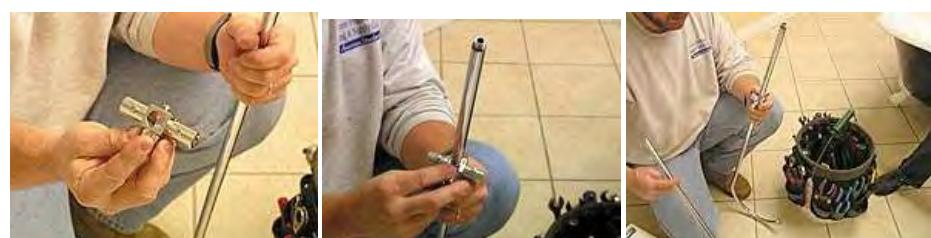
16. Screw in the 2nd part of the riser pipe to the shower head pipe.
