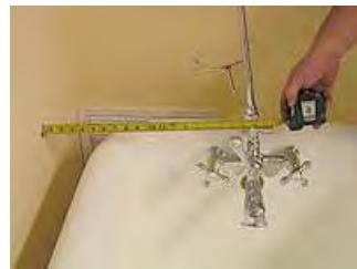
27. Hold the escutcheon at the measurement from 26 to mark the two holes with a pencil.
