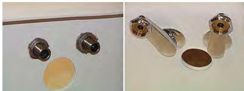
7. To attach the faucet body to the swing arms you will need to take the lock nut washer and install in the lock nut.
