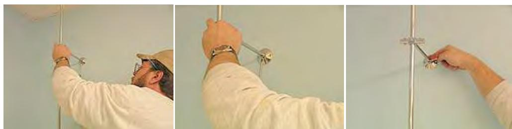
32. Level the post and tighten the front set screw.
