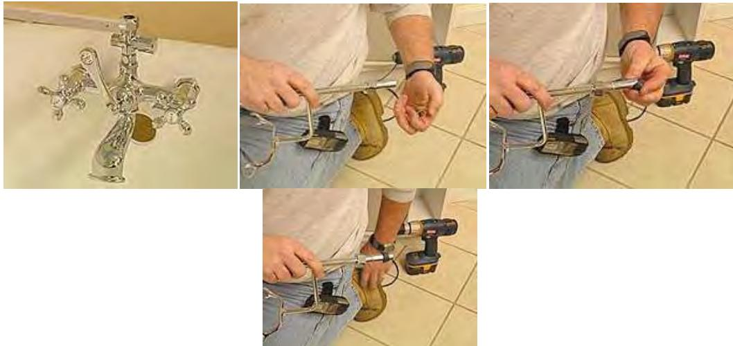
19. Screw the locknut at the bottom of the riser pipe to the faucet body. (Note: if the cone washer included is too big, then have the plumber switch it with a smaller cone washer or shave it down to the correct size)
