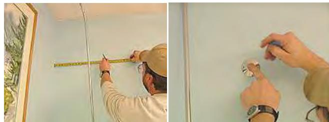
28. Use the power drill to drill holes (Note:  $\frac{1}{4}$ " drill bit is required)
