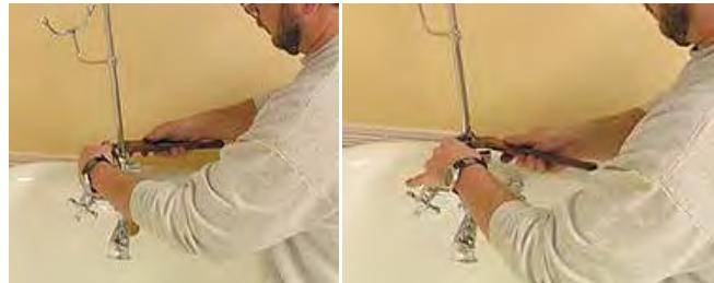
21. Measure from the wall to center of the diverter valve.
