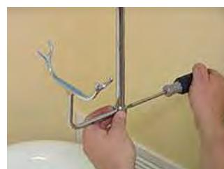
34. Screw the hose to the diverter valve and set the hand shower on the cradle.
