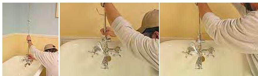
20. Use the pipe wrench to tighten the locknut.
