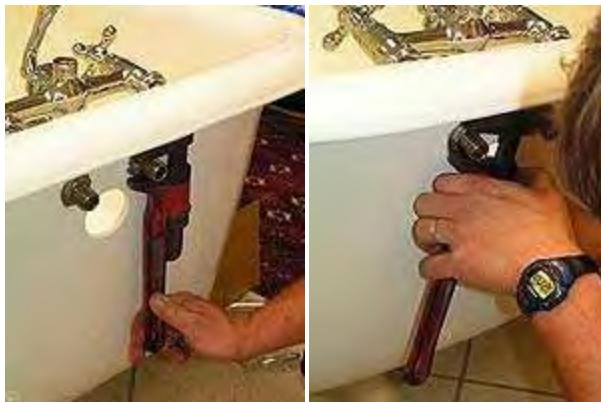
13. Place the cone washer into the shower opening. Screw the diverter valve into shower opening.
