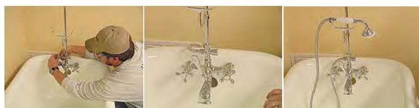
35. Use channel locks to tighten the hose locknut.
