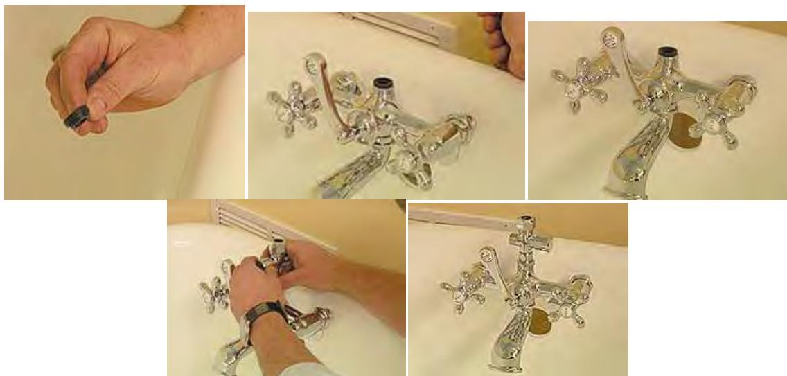
14. Use the pipe wrench to tighten the lock nut.
