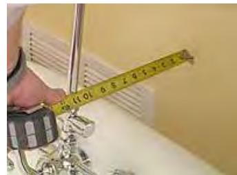
22. Use the measurement from step 21 to measure from the wall to the center of the pipe.
