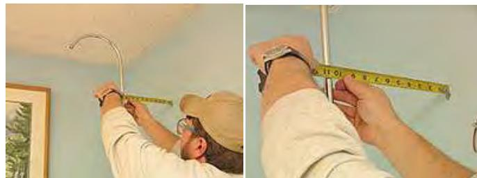
23. Take this measurement and subtract  $\frac{1}{2}$ " (this is to incorporate the distance of the center to the thread of the bracket).
