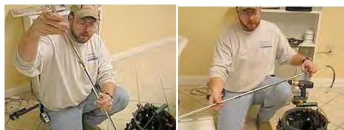
17. Place the arm for the hand held shower onto the riser pipe.
