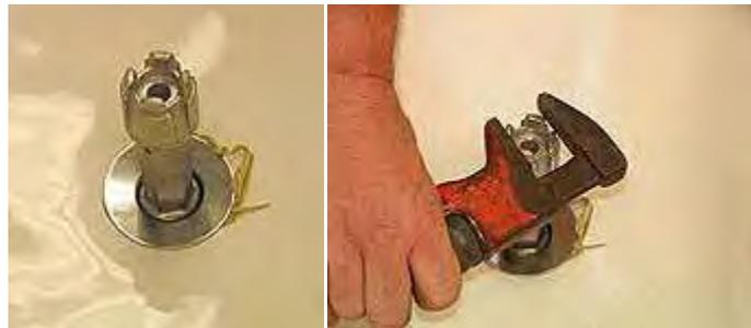
10. At the end of the connecting pipe, slide the lock nut onto the pipe first and then slide the 1 3/8" trap washer. (Please note: the grooved end should always be to the "T" connection, as shown). Prior to cutting tubes to size; overflow, waste tube and tailpiece should be seated to ridge inside "T" to size it correctly and make a proper leak free connection.
