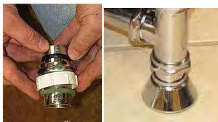
17. Apply a liberal amount of thread sealant on the threaded area of the overflow tube. (Use teflon tape instead of thread sealant if the finish is supercoated brass.)
