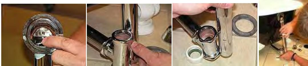
21. You will then use a 1 1/2" tubing cutter to cut the pipe.
