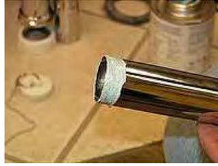
18. Screw the overflow receiver to the overflow tube.
