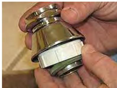
15. Slide the escutcheon onto the tailpiece which will cover the rough in to the floor.
