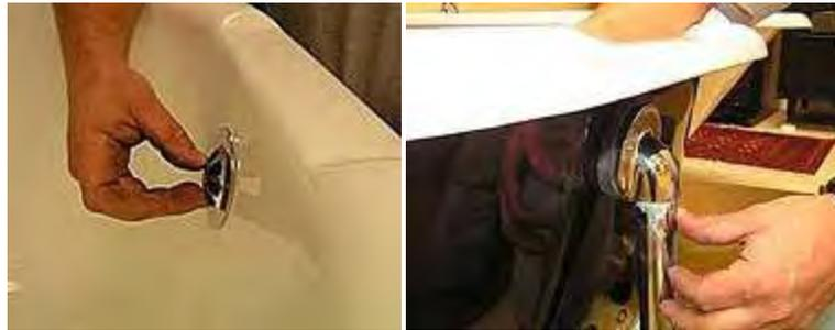
25. Begin turning the screw into the overflow receiver. If the screw is too long, you will need to measure any excess amount by making sure the screw is all the way in and the overflow plate is pushed onto the tub.
