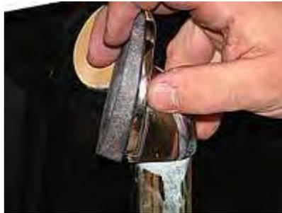
24. Place the overflow cover onto the front hole and place the overflow receiver on the back of the overflow hole.
