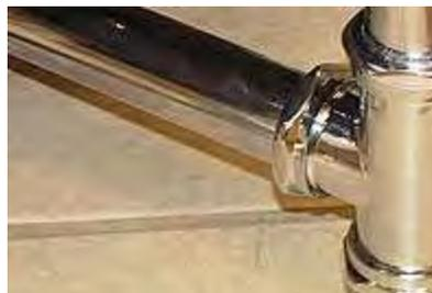
12. To obtain a cutting measurement for the tail piece you will need to determine the length from your trap adaptor to the "T" (Example images of trap adaptors you may have in your home are pictured below).
