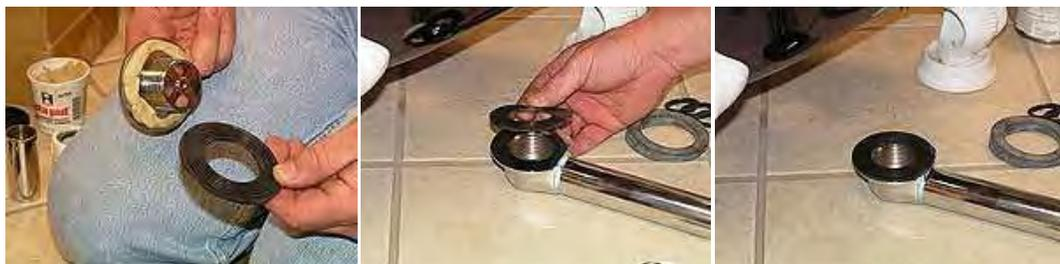
8. Hold the shoe to the bottom of the drain hole and the PO plug to the top of the drain hole and begin to screw using the PO plug wrench.
