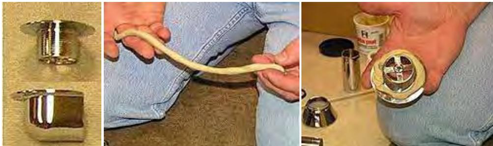
7. Take the PO plug washer with the ribbed side facing up and place it on top of the shoe.
