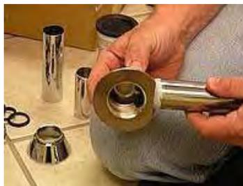
4. Apply the strap wrench to the pipe and attach the smooth jawed pipe wrench to the shoe to assist with hand tightening a 1/4 turn. (Please note: over tightening will strip the threaded area.)
