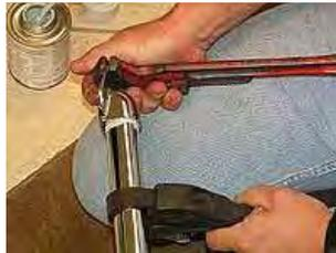
20. To obtain the cutting measurement you will start measuring from the center of the overflow receiver to the farthest point the tube will fit inside the "T" and place a mark on the tube.
