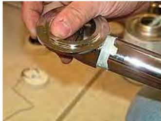
19. Apply the strap wrench to the overflow tube and attach the smooth jawed pipe wrench to the overflow receiver to assist with hand tightening a 1/4 turn. (Please note: over tightening will strip the threaded area.)
