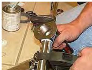
5. Place the shoe onto the bottom of the drain hole. Place the "T" above the trap adaptor to get an accurate measurement. Place the connecting pipe against the "T" and mark the pipe where the arrow indicates below. Use a 1/2" pipe cutter to cut down the pipe.
