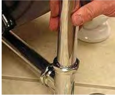
23. Place the beveled overflow washer onto the overflow receiver. (Please note: the wider end of the washer is always towards the floor.)
