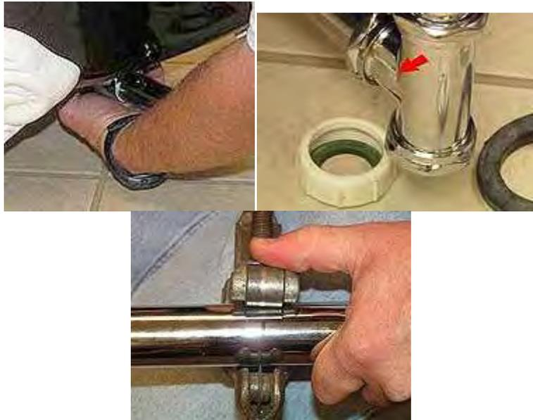
6. You will then unscrew the PO plug from the shoe. Take plumber's putty and roll it 3/8" thick and apply it to the PO plug. (Please note: plumber's putty is not to be used on supercoated brass. The manufacturer recommends a bead of silicone.)
