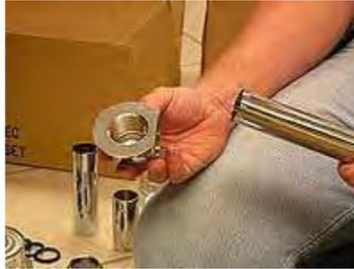
2. Apply a liberal amount of thread sealant to the threaded area on the connecting pipe.
