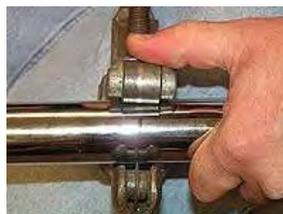
22. Slide the lock nut onto the overflow pipe first and then the trap washer and connect to the "T".
