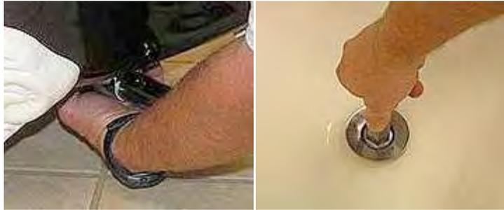
9. Place the PO plug wrench into the PO plug and use the smooth jawed pipe wrench to hand tighten a 1/4 turn.
