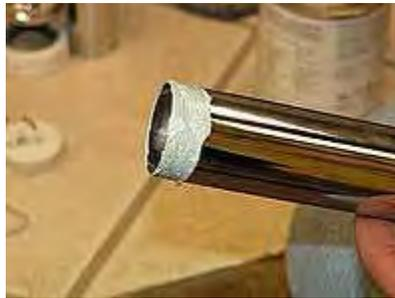
3. Screw the shoe onto the connecting pipe.
