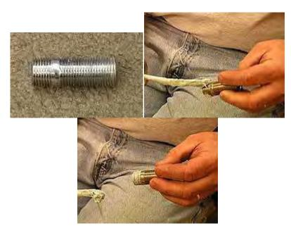
2. Tighten the faucet nipple to the 1/2" thread on the faucet swing arm. You want to hand tighten a 1/4 turn using the strap wrench.
