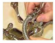
17. Use the strap wrench to tighten the hose lock nut.
