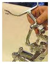
15. Use the smooth jawed pipe wrench to tighten lock nut. Turn until tight.
