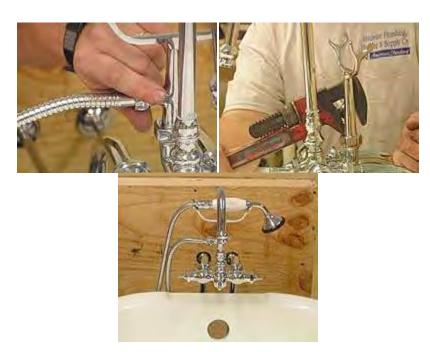
26. For handle attachments, remove screws from the faucet body valves (handshower diverter, Hot and Cold) (Note the red washer for hot, blue washer for cold) and attach appropriate handles with screws.
