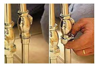
19. Tighten wall bracket ring to wall nipple/brace.
