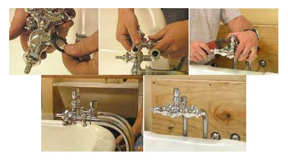
21. Thread sealant applied to spout and hand-tighten into faucet body.
