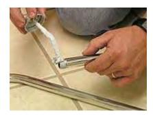
4. Tighten valve end with o-ring to valve nipple.
