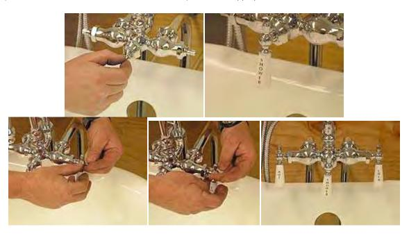
27. Do the same for the Hot and Cold shut off valves located toward the bottom of the supply lines.
