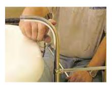
17. Assemble valve and supply line to wall bracket.
