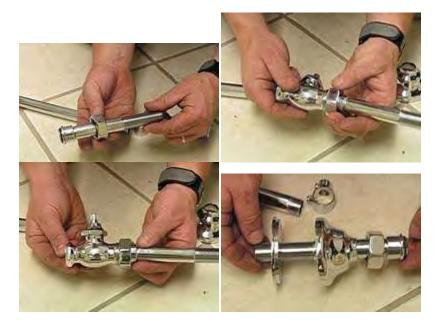
7. Using allen wrench tighten valve assembly to rough in and tighten with allan wrench into floor.
