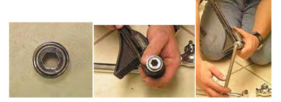
6. Slide valve lock nut onto assembly facing where valve will attach then slide escutcheon and floor plate onto assembly as shown.
