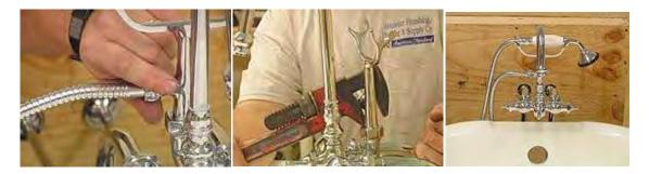
26. For handle attachments, remove screws from the faucet body valves (handshower diverter, Hot and Cold) (Note the red washer for hot, blue washer for cold) and attach appropriate handles with screws.
