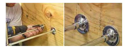
16. Note: No specific height for wall bracket except that it has to be below the bend and above the valve.
