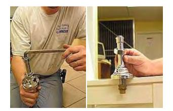
8. Slide wall bracket ring up the supply line.
