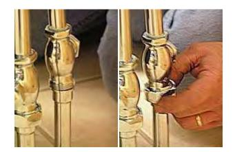
19. Tighten wall bracket ring to wall nipple/brace.
