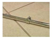
9. Add thread sealant to valve side of thread and attach valve to supply and tighten with strap wrench and smooth jawed wrench.
