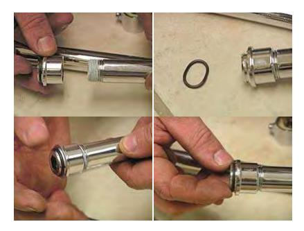
5. Place allen wrench into allen opening and strap wrench to tighten valve end to nipple until tightened.
