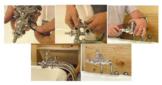
21. Thread sealant applied to spout and hand-tighten into faucet body.
