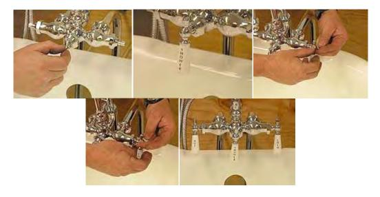
27. Do the same for the Hot and Cold shut off valves located toward the bottom of the supply lines.
