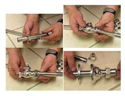
7. Using allen wrench tighten valve assembly to rough in and tighten with allan wrench into floor.
