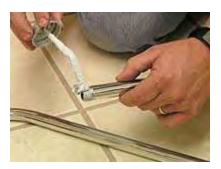
4. Tighten valve end with o-ring to valve nipple.
