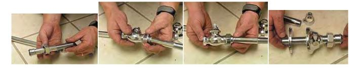
7. Using allen wrench tighten valve assembly to rough in and tighten with allan wrench into floor.
