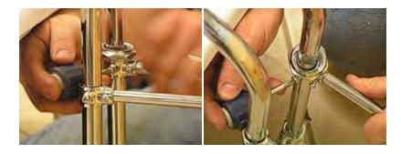
20. Hand tighten lock nut washer on supplies to faucet and tighten a 1/4 turn.
