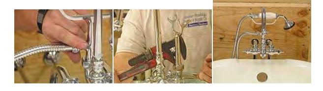
26. For handle attachments, remove screws from the faucet body valves (handshower diverter, Hot and Cold) (Note the red washer for hot, blue washer for cold) and attach appropriate handles with screws.
