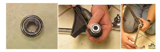
6. Slide valve lock nut onto assembly facing where valve will attach then slide escutcheon and floor plate onto assembly as shown.
