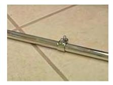
9. Add thread sealant to valve side of thread and attach valve to supply and tighten with strap wrench and smooth jawed wrench.
