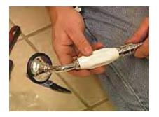
25. Attach small lock nut side of hose into cradle inlet. Hand tighten a 1/4 turn using the smooth jawed pipe wrench.
