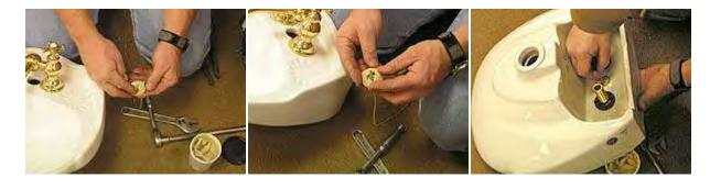
9. Place the metal break and screw the lock nut onto the chain stay screw with an adjustable wrench.
