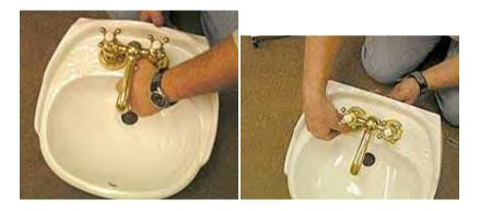
8. Place plumber's putty on the chain stay and insert the chain stay in the hole.
