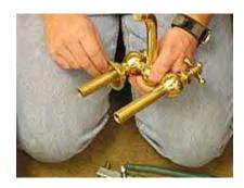
2. Place ¼" bead of plumber's putty on the bottom of both escutcheons. This will create a seal between the faucet and the sink.
