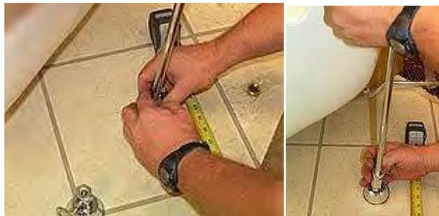
Screw the lock nut at the top of the supply line to the faucet nipple
