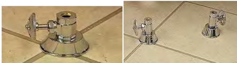
4. To attach the supply lines you will first need to measure the length. In order to find out this measurement you will need to measure from the floor to the center of the faucet nipple.
