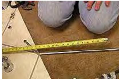
8. Use a  $1/2"$  tubing cutter to cut to size.
