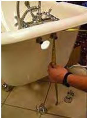
5. Then measure from the floor to the top of the compression nut. From this measurement you will want to subtract  $1/2"$  (this measurement is the depth of the compression fitting).
