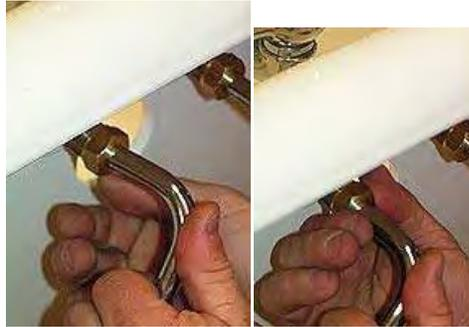
13. Hand tighten the lock nut a 1/4 turn using the smooth jawed pipe wrench.
