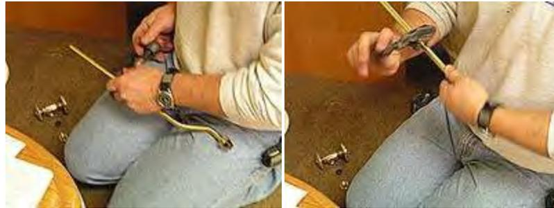
12. Place the lock nut and washer on the end of the supply line and screw into the shut off valve.
