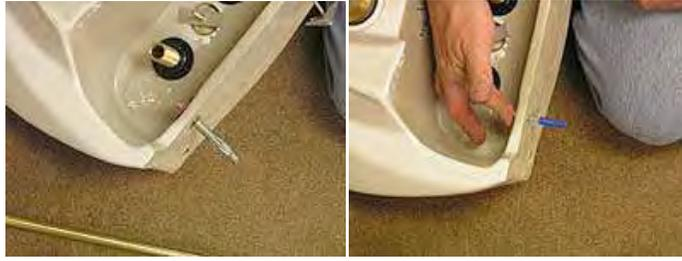
6. Place the sink on the pedestal base making sure the toggle bolts go into the 7" mounting holes in the wall.
