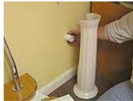
2. Shut off valves will be located 3 1/4" distance from locknut to finished wall and 21" from the floor to the center of the shut-off valves. (This measurement is product specific)
