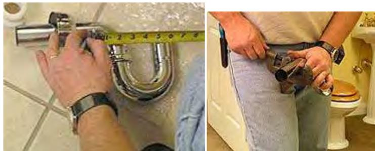
17. Tighten the 3 trap locknuts using the channel locks.
