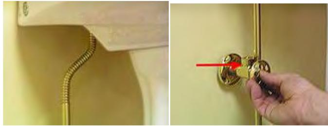
11. Mark this measurement on the supply lines and use a 1/2" tubing cutter to cut the supply lines.
