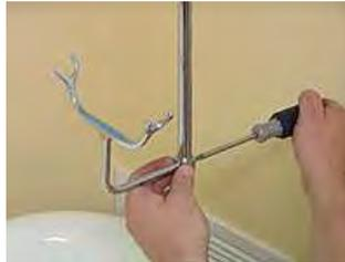
22. Screw the hose to the diverter valve and set the hand shower on the cradle.
