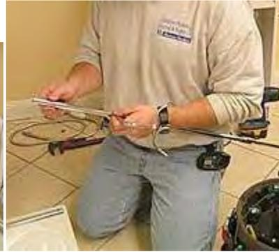
6. Take the locknut from the diverter valve and place it at the bottom of the riser pipe. Slide the friction ring and washer onto the bottom of the riser pipe.
