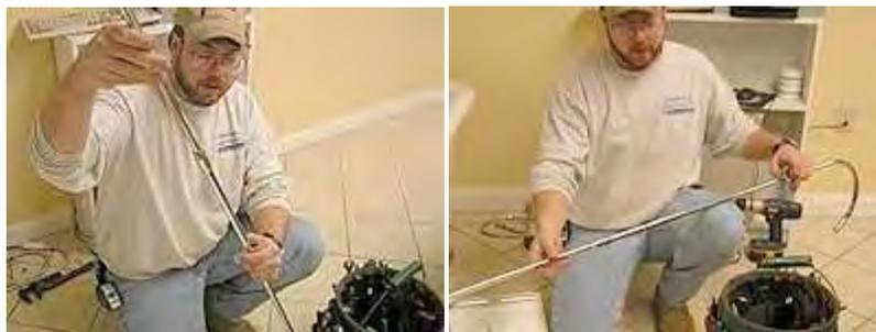
5. Place the arm for the hand held shower onto the riser pipe.
