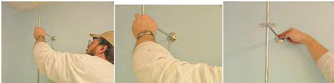
20. Level the post and tighten the front set screw.
