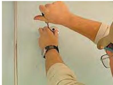
19. Slide the post into the bracket and tighten the set screw.
