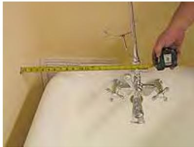
15. Hold the escutcheon at the measurement from 14 to mark the two holes with a pencil.
