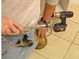
7. Screw the locknut at the bottom of the riser pipe to the faucet body. (Note: if the cone washer included is too big, then have the plumber switch it with a smaller cone washer or shave it down to the correct size)
