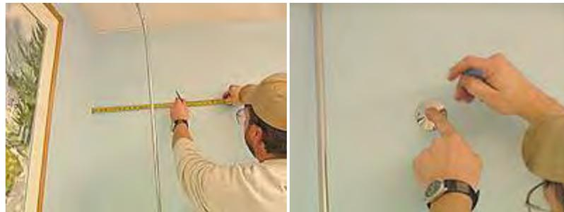
16. Use the power drill to drill holes (Note: 1/4" drill bit is required)
