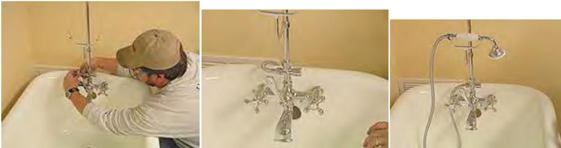
23. Use channel locks to tighten the hose locknut.
