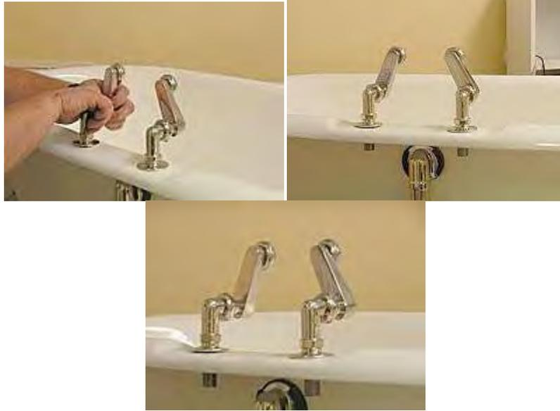
10. Hand tighten the lock nuts to the faucet body.
