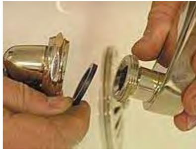
8. Tighten the lock nut to the swing arm. Hand-tighten a 1/4 turn using strap wrench.
