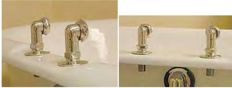
7. Take the lock nut washer and install in the lock nut to attach the modified swing arm to the deck mount coupler.
