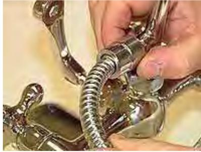
18. Use the strap wrench to tighten the hose lock nut.
