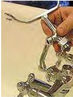
16. Use the smooth jawed pipe wrench to tighten lock nut. Turn until tight.
