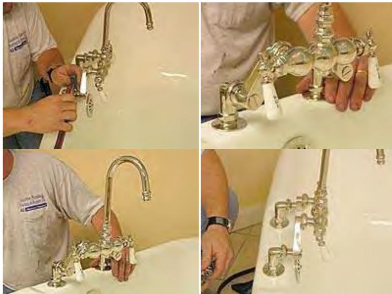
14. To attach the handshower holder, attach the washer to the lock nut.
