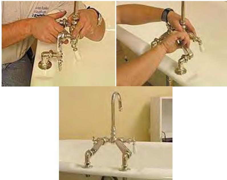
11. Apply the smooth jawed pipe wrench to the lock nut and tighten a 1/4 turn.
