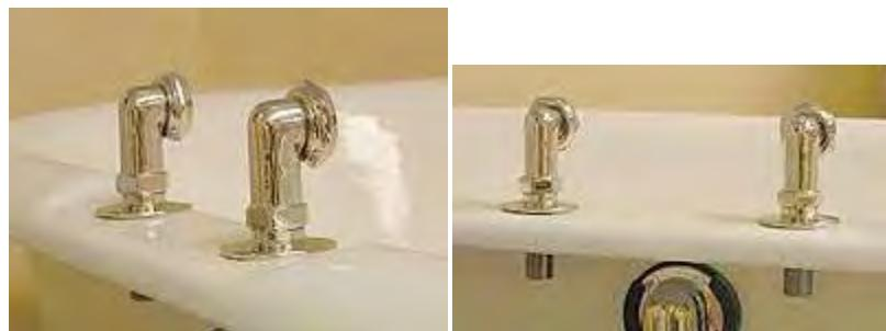
10. Take the lock nut washer and install in the lock nut to attach the modified swing arm to the deck mount coupler.
