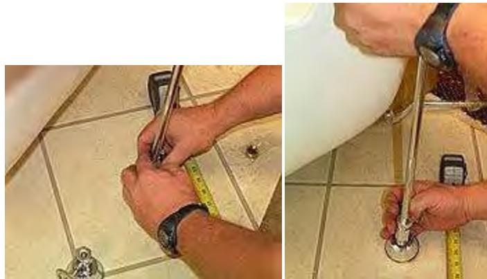
26. Using the smooth jawed pipe wrench, screw the lock nut at the top of the supply line to the faucet nipple.
