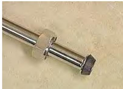
23. Remove the compression lock nut from the shut off valve. Slide the compression lock nut, the friction ring (make sure to choose the right size), and the supply washer (make sure the beveled end is facing towards the faucet) to the bottom of the supply line.
