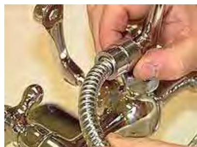
33. Use the strap wrench to tighten the hose lock nut.
