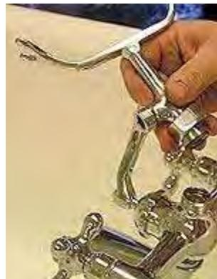
31. Use the smooth jawed pipe wrench to tighten lock nut. Turn until tight.
