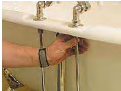
27. Hand tighten the lock nut a 1/4 turn using the smooth jawed pipe wrench to tighten the lock nut.
