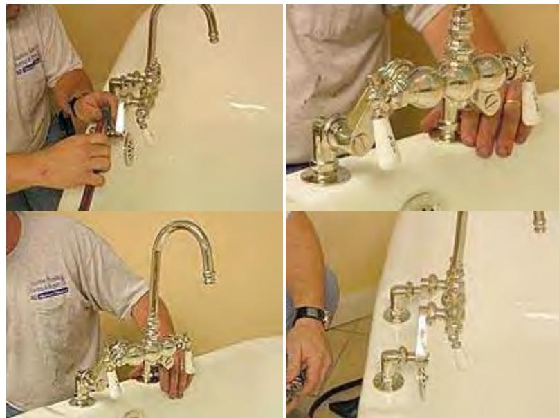
17. To attach the supply lines, you first need to measure the length. In order to find out this measurement, you will need to measure from the floor to the flat bottom portion of the faucet nipple.
