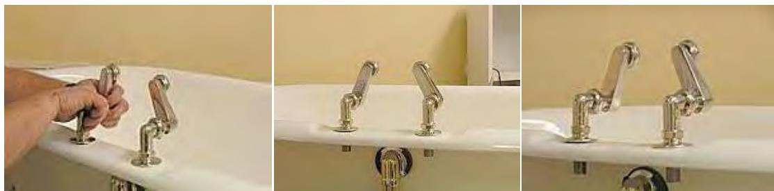
13. Hand tighten the lock nuts to the faucet body.
