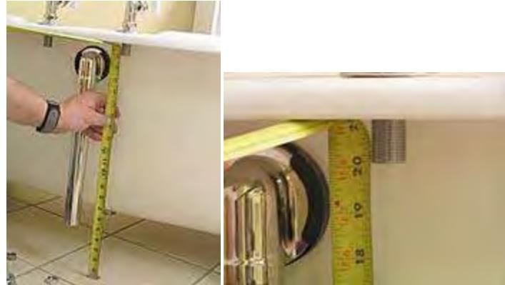
18. Then measure from the floor to the top of the compression nut. From this measurement you will want to subtract 1/2" (this measurement is the depth of the compression fitting).
