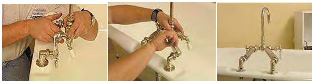
14. Apply the smooth jawed pipe wrench to the lock nut and tighten a 1/4 turn.
